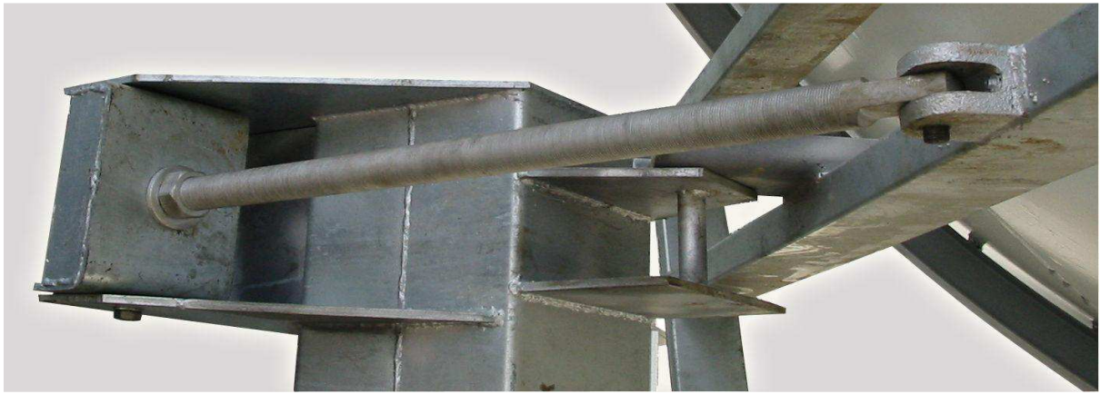
Picture 07 – Azimuth Adjustment Axle
