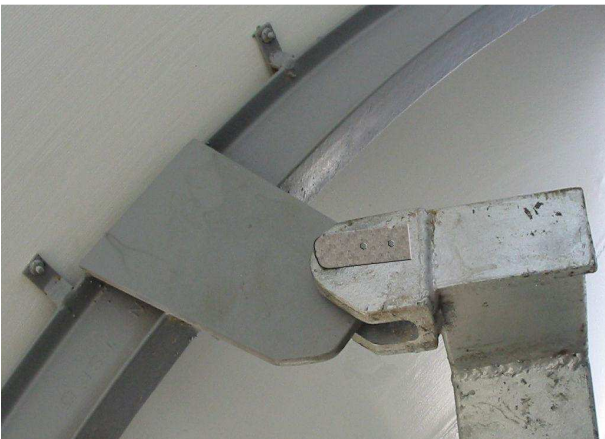
Picture 10 – Reflector's connection to mount.
